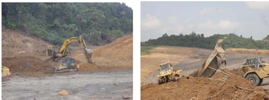
Fig. 1. Topsoil stripping and placement
