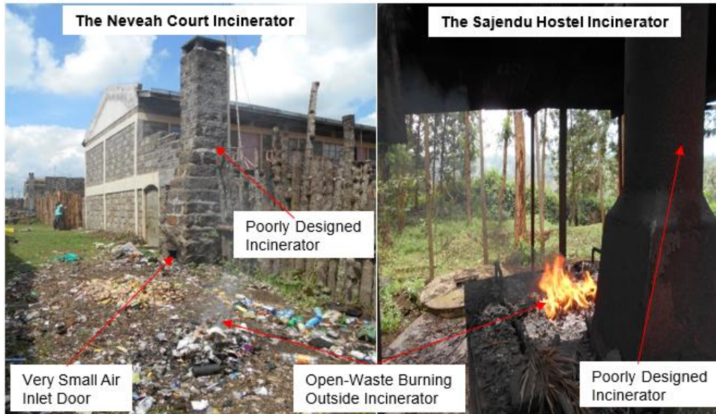
Fig. 6. The poorly designed incinerators resulting to open-waste burning
